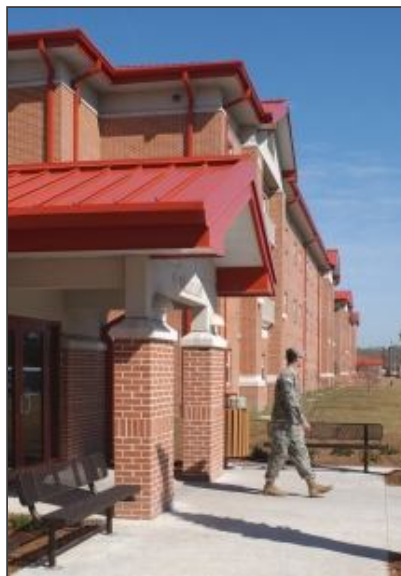
The Savannah District of the U.S. Army Corps of Engineers recently built new barracks for Rangers at Hunter Army Airfield. Photo by USACE
