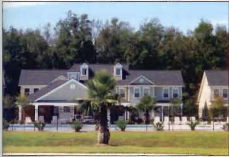
Independence already has a 260-unit apartment complex and a townhome community available for occupancy.
